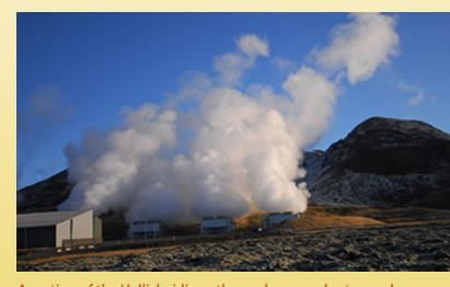
A section of the Hellisheidi geothermal power plant complex. Courtesy Creative Commons by Martin V. Morris; Licensed under CC BY-SA 2.0. Hellisheidi, the newest and largest geothermal project in Iceland, is a flash steam plant that can generate 300 MW of power and 400 MW thermal.
