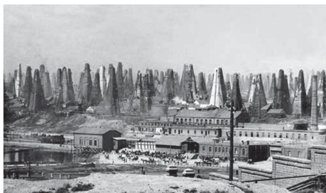
The Nobel brothers oil wells in Balakhani close to Baku. The tightly spaced derricks were fire hazards and the noise levels were described as “horrendous.” Photo courtesy of Asbrink Collection and Petroleum History Institute.
